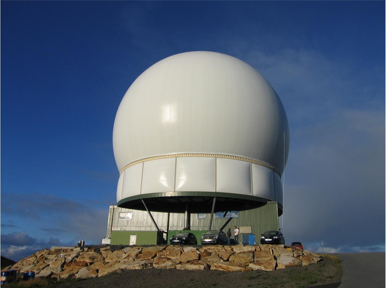
**GLOBUS II is pictured above. GLOBUS II a radar system located at Vardo, Norway, that is operated solely by Norwegian personnel, but which was developed by the United States and serves as part of the 29-sensor, global space surveillance network that provides data to the US Strategic Command. Engineers from AFRL/RX recently made a trip to Norway to perform thermography inspections on the radar.**
