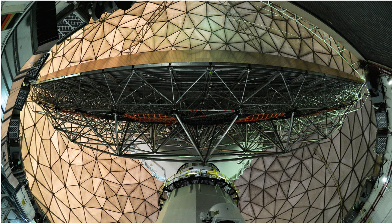
FIGURE 14. Only a few inches of clearance exist between the edges of the reflector and the space frame of the radome; as a result, the photographer resorted to a fisheye lens to capture the completed HUSIR antenna in its entirety, as shown above. The photograph was taken during a ribbon-cutting ceremony held on 11 February 2014 at the Lincoln Space Surveillance Complex to welcome HUSIR to the U.S. Space Surveillance Network.
